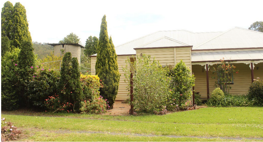
Figure 10: Southern façade showing recent additions to left of image, with the original veranda configuration and hipped roof form (right of image). Note the position of the silo to far left.
