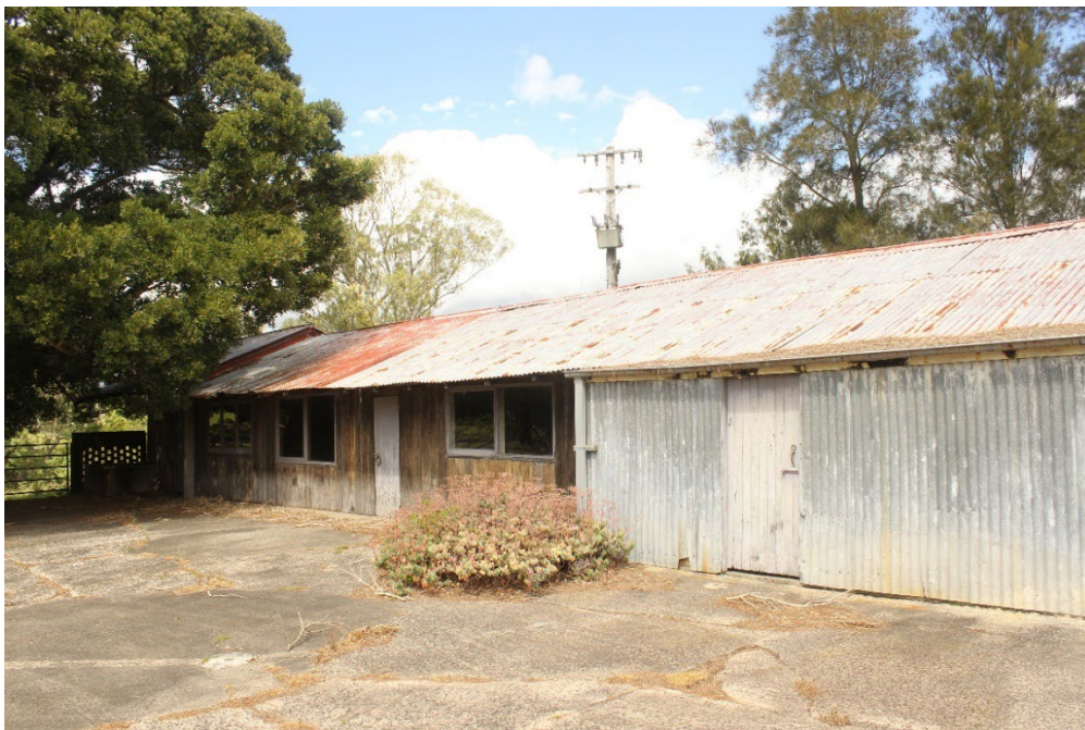
Figure 14: Eastern façade of dairy showing phased construction, modifications and recladding.
