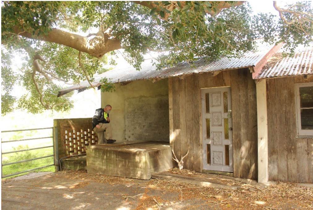
Figure 12: Southern end of dairy building, showing raised milk storage area and recent vertical slab cladding (recycled bull pen fencing) and residential door which were added to the building during the 1990's modifications.
