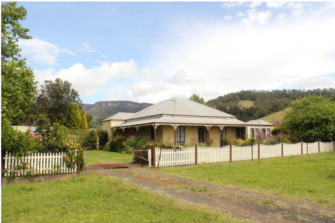
Figure 21: Miala showing the picket fence and garden setting of the house with escarpment backdrop behind. Note the cattle grate to the entry.
