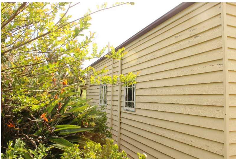
Figure 9: Western Façade of Miala. This elevation was modified in the 1990's additions and adaptations and does not represent significant fabric.
