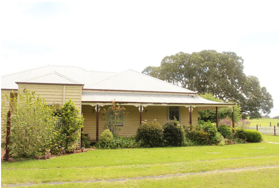
Figure 11: Southern façade of Miala cottage showing original veranda detail and original intact hipped roof form (right of image) and additions (left of image). Note the large established Fig.
