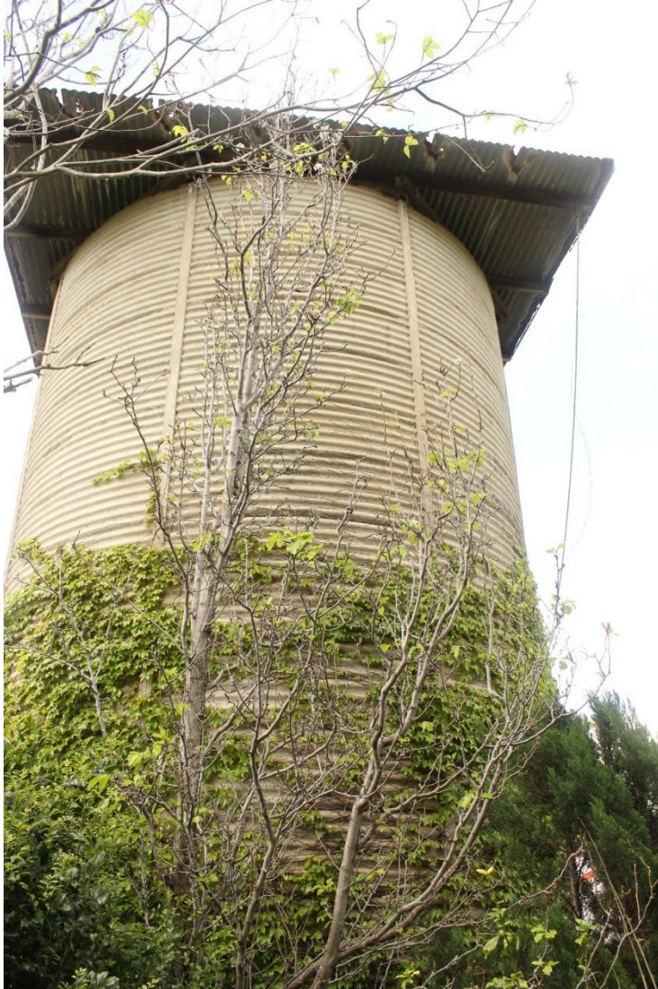
Figure 17: Detail of corrugated concrete silo located to the north west of the house. The flat roof structure tied to the ground with wires.
